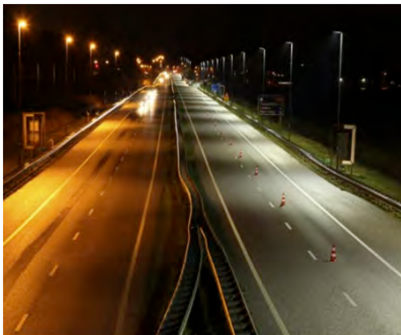
Figure 1. LED streetlight installation (right) adjacent to HPS installation (left) [source: http://homelights.blogspot.ca/2011_04_01_archive.html ]
