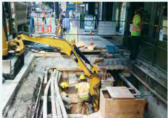
City carpenters working on Fort Street.
