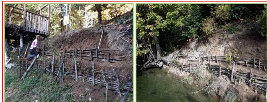
Figure 7. Construction of a live-stake wattle fence at two CSSP 2018 sites along Cowichan River
